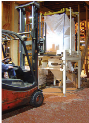
Top section being lowered on to discharger base
