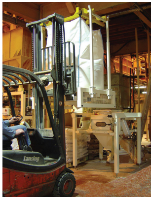
Top section complete with bulk bag being returned to the discharger
