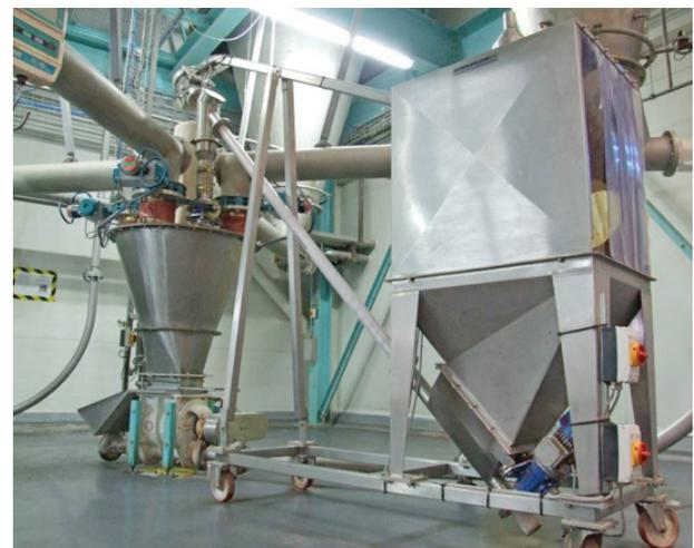
Cocoa powder being conveyed to mixer with Spiroflow's Flexible Screw Conveyor
