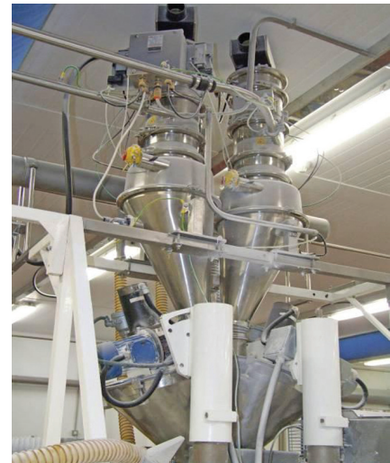
The vacuum transfer system to the packing machines
