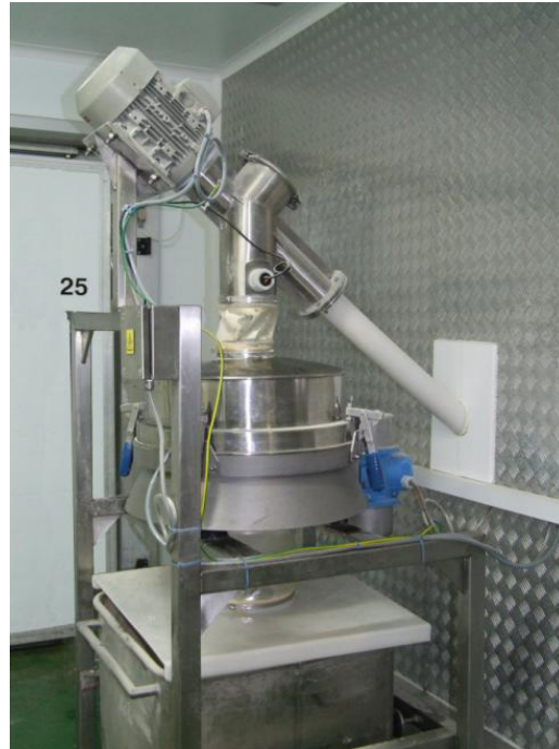
Outlet of Flexible Screw Conveyor discharging bread crumbs via a sifter in to tubs in the production area
