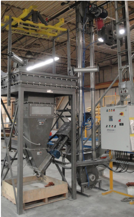
Cement powder is unloaded with the T4 Bulk Bag Unloader, moved out of the hopper with Dual Flexible Screw Conveyors to a vertical Aero Mechanical Conveyor.
