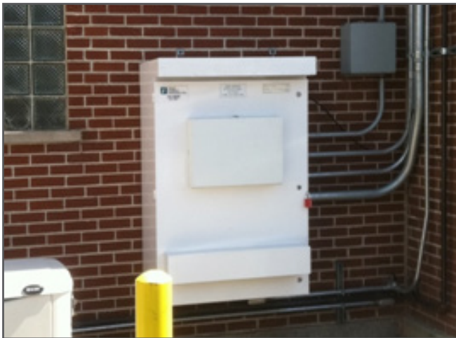
Remote I/O panels were installed near sensors in each production area.
