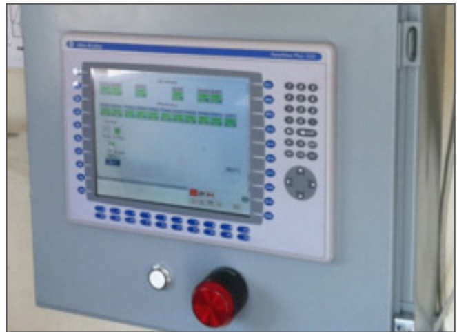
Remote I/O panels were installed near sensors in each production area.
